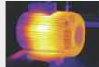
Motor: Internal Winding Problem
