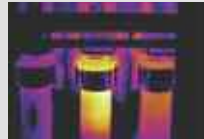
Electrical: Hot Fuses
